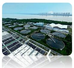
A wastewater treatment project located in coastal city of Eastern China. The project consists of 128.71 km and 173.44 km of a new-built and a renovated sewage pipeline system respectively. The annual sewage treatment capacity of the project is 72 million tons. The Bank's loan accounted for approximately 59.79% of the total project investment, which reduced COD by 23,246 tons/year and NH<sub>3</sub>-N by 4,090 tons/year.
